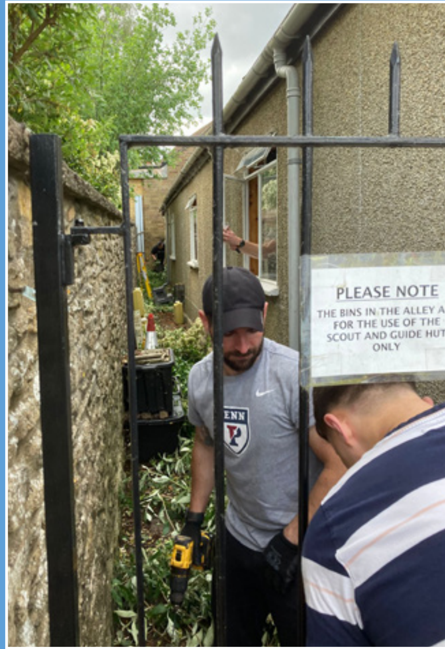
Chris and Chris repairing the fence whilst Jon is cutting back the overhanging branches
